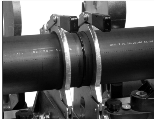
Cooling the weld seam
