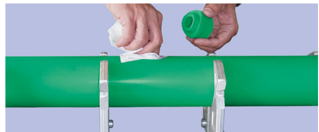
② Clean the hole, degrease the fitting and drill a hole.
