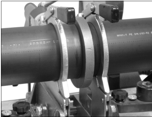
Heating with the heating plate
