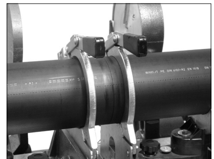
Properly prepared for welding
